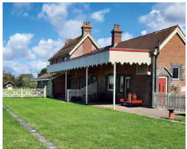
Whitwell Station has been sympathetically converted into two self-catering cottages.
