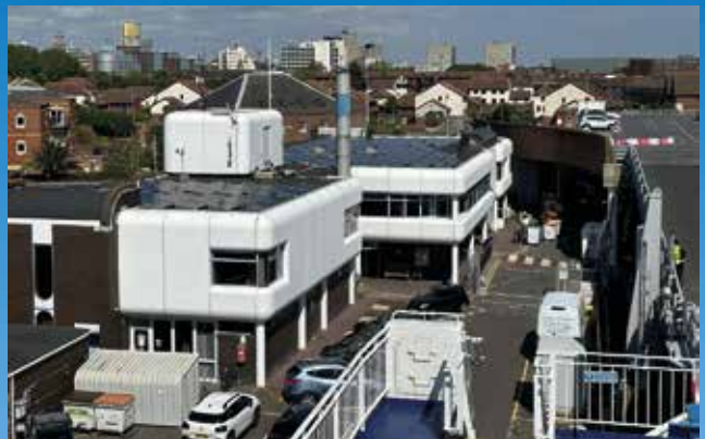
Solar panels have been installed at our port in Gunwharf Road Portsmouth
